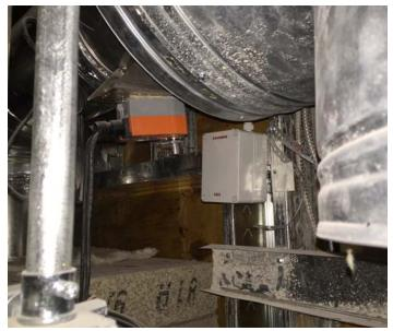
ENERVEX's Automatic Damper (ADF) and Pressure Sensor (XTP)
