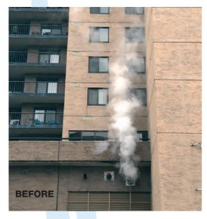
The exhaust plume is creating ice build-up and potential deterioration on the wall. And is a nuissance to the residents.
